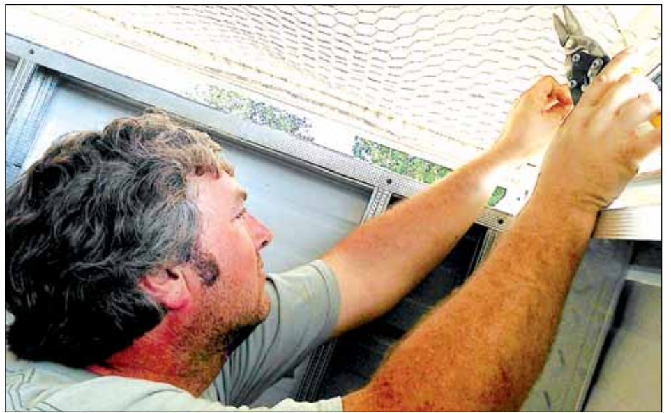
Ken Clark installs chicken wire between the church walls and roof.
