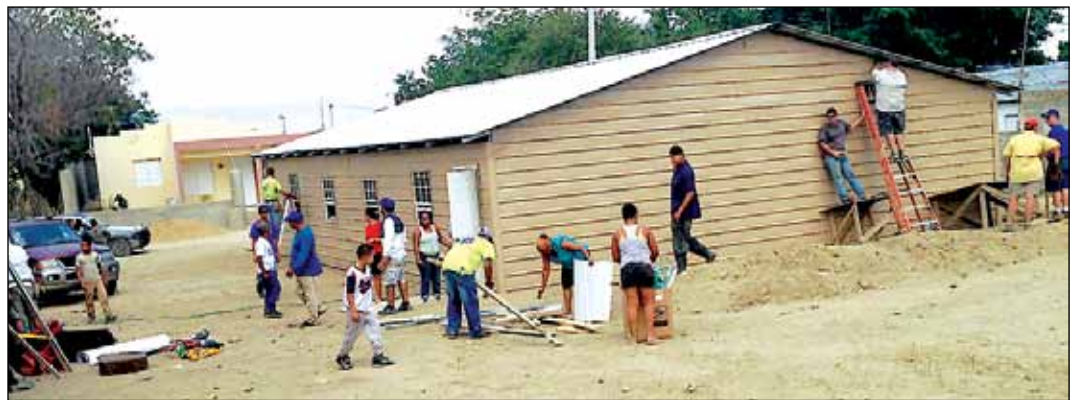
Finishing touches are put on the church.
