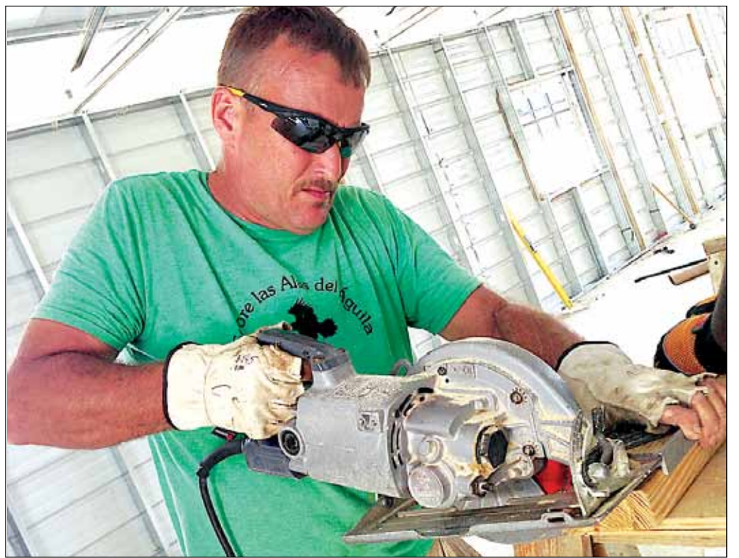
Neal Turner cuts lumber for final details.
