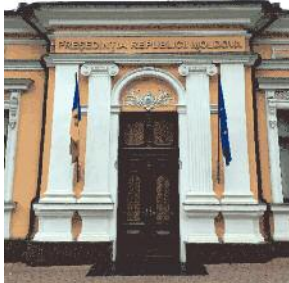
The Presidential building in Chișinău, made of concrete.
