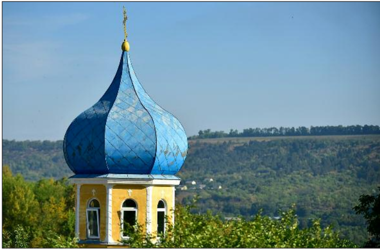
A dome atop the monastery in Calaraseuca in northeastern Moldova.
